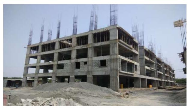
In Block C2: Second Floor level Slab 2<sup>nd</sup> half Shuttering & Bar bending work in progress.
