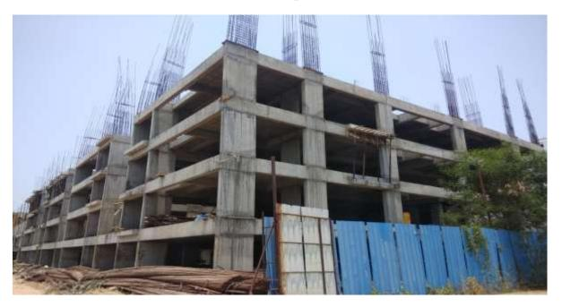
In Block D3: First floor Column Shuttering and Bar bending Works in Progress.
