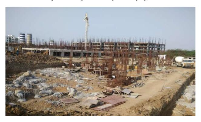
In Block A2: Pile Cap & Plinth Barbending work on progress.
