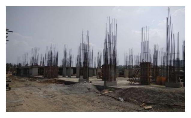
In Block D1: Excavation, Bar bending & Shuttering for Pile cap work on Progress.
