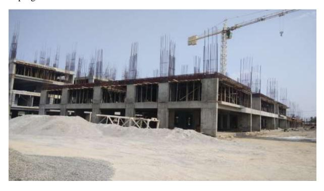
In Block C3: First Floor level Slab  $1^{st}$  half Concrete completed . Shuttering & Bar Bending Work for columns on progress.
